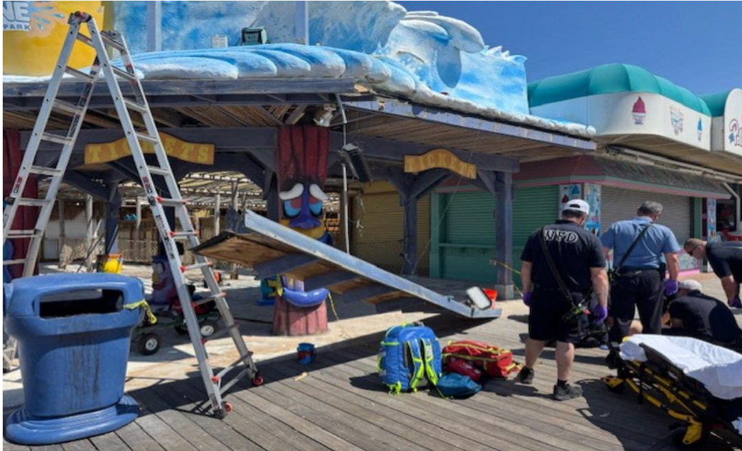
Roof Collapse 3500 Boardwalk 6/2/2025
